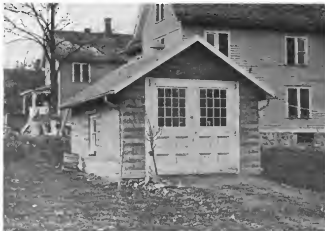
Cement Block Garage for One Car Is Low In Cost
